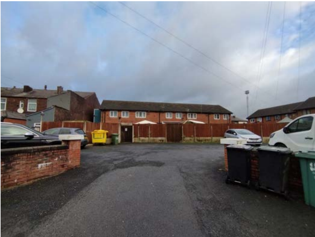
Photo 2 – Rear elevation across car park
